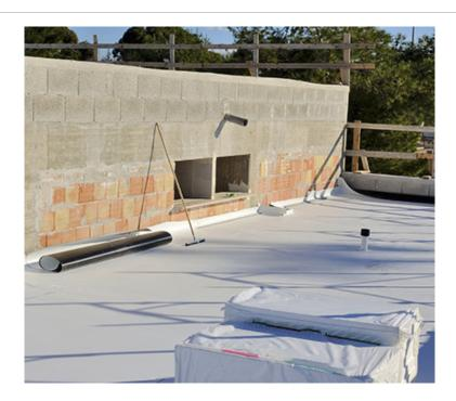
Stadium construction was centred in an area where the level of the water table was high, which involved both careful planning and organisation of the site. Water with a high-variable degree of hardness – and also containing salts and other particularly aggressive chemical products – may come in contact with stadium construction; this requires the use of an advanced waterproofing system.
